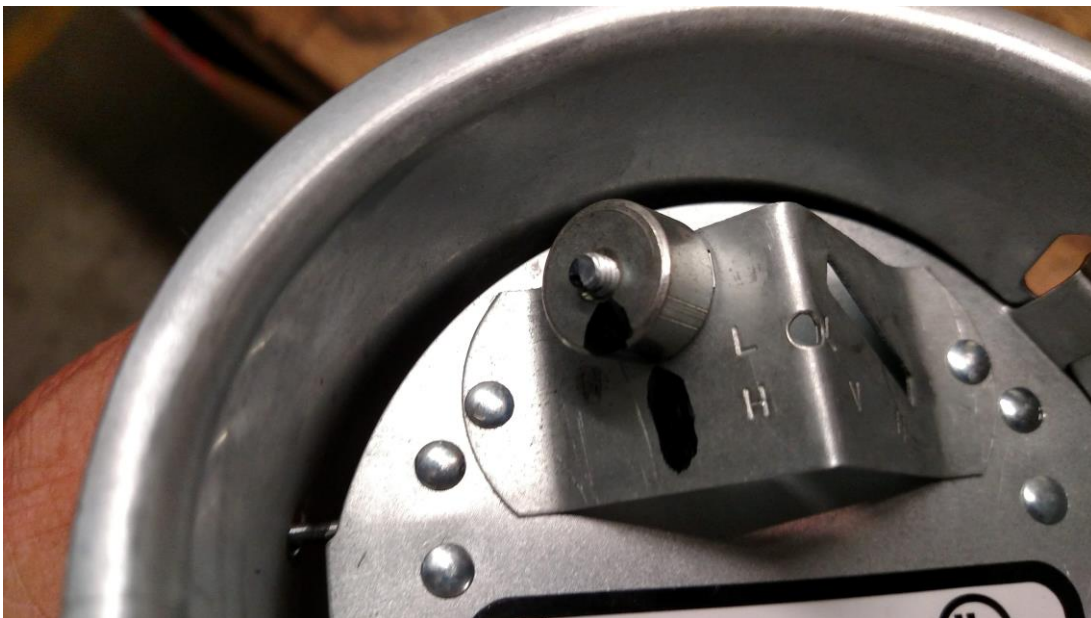
FIGURE 3 WEIGHT LOCATION FOR HORIZONTAL DIRECT VENT
